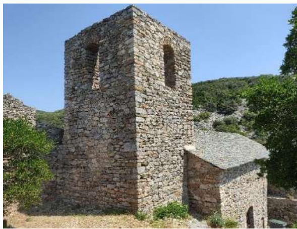
Figure 71. Chapelle Castrale de Cabrerolles
